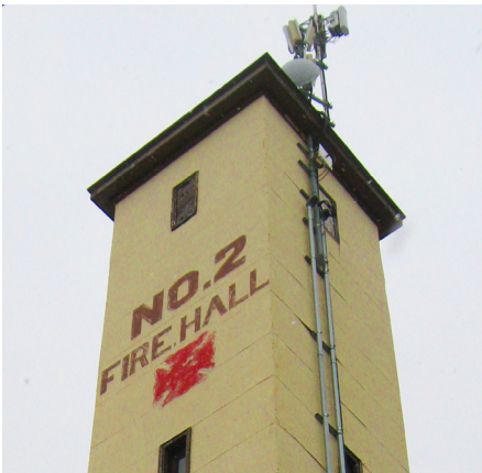
FIGURE 5. FIRE DEPARTMENT HOSE DRYING TOWER FOR BASE STATION
