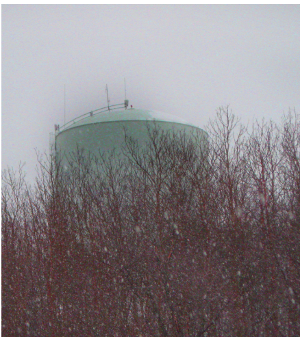
FIGURE 6. WATER TOWER FOR BASE STATION
