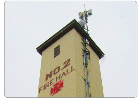
Fire department hose drying tower for base station
